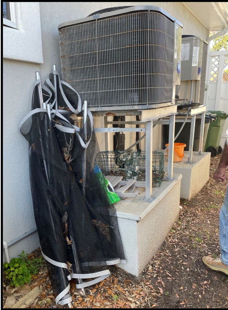
❖ Elevate Mechanical/ Electrical Equipment
