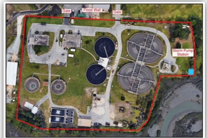
Figure 10: Perimeter Flood Wall and Pump Station
