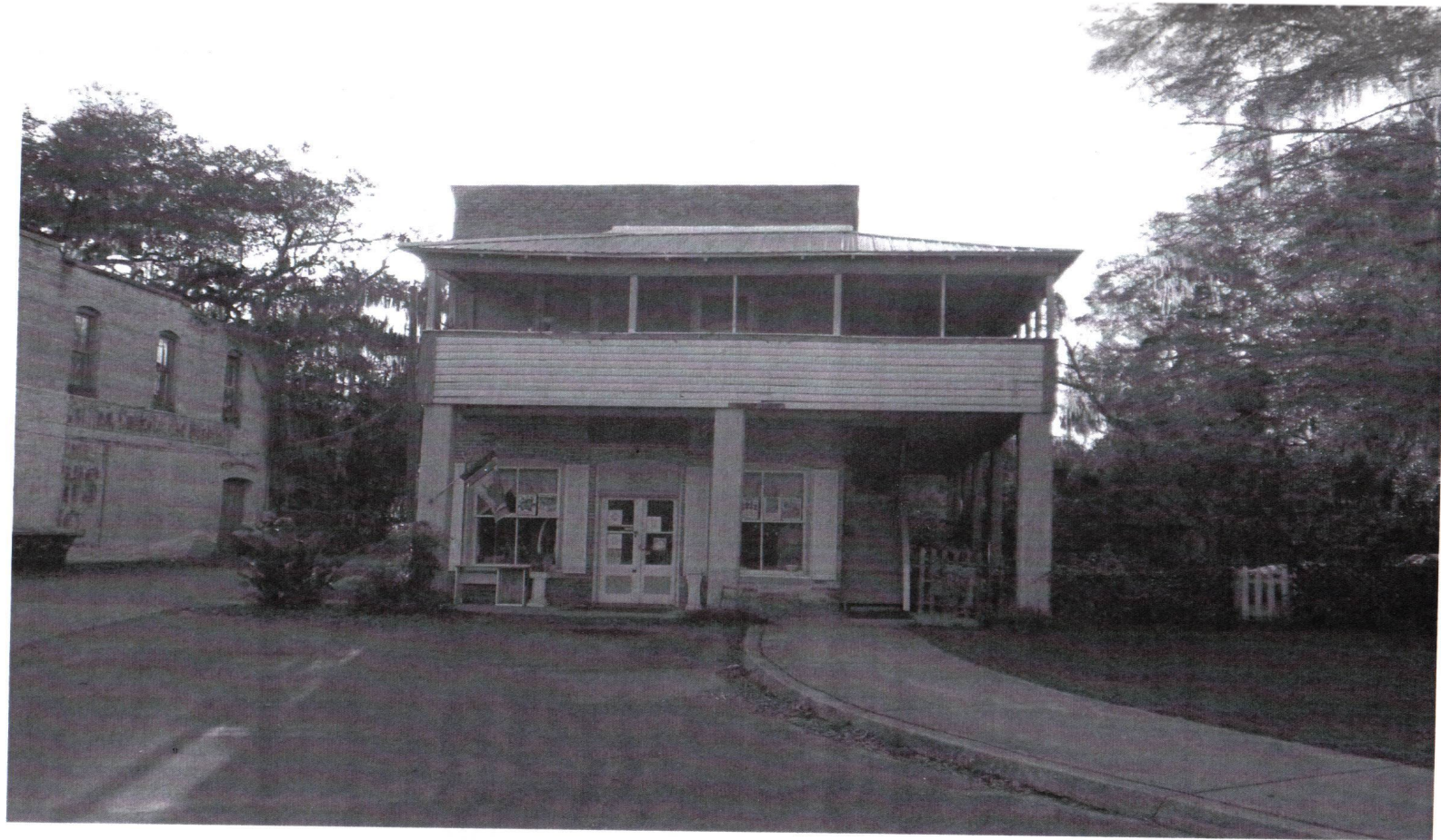
AL2353-SMITH BUILDING-302 NE 1 ST STREET
